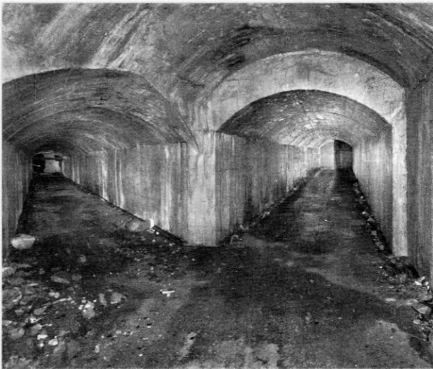
Laye Tunnel - Intersection of the two entrance tunnels
